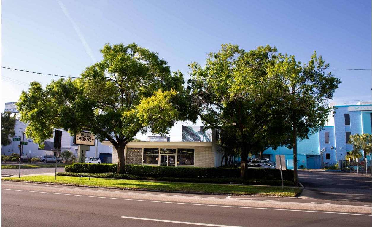
1900 First Avenue North will be the new home to St. Pete Eye Care Specialists. (Photo by Vector Commercial Real Estate)
